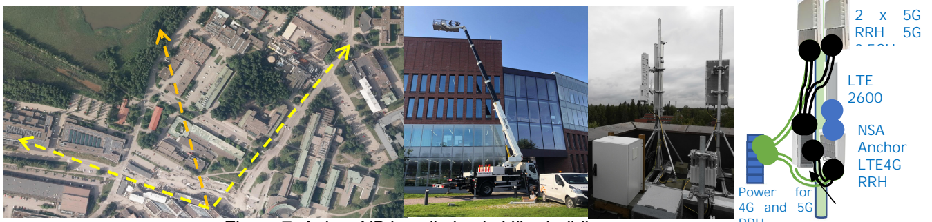
Figure 7. Aalto gNB installation in Väre building.
